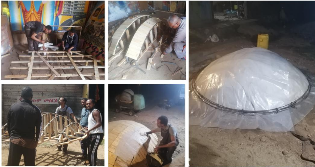
Formwork assembly and surface finishing
