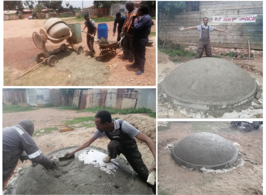
Prototype concrete mixing and casting
